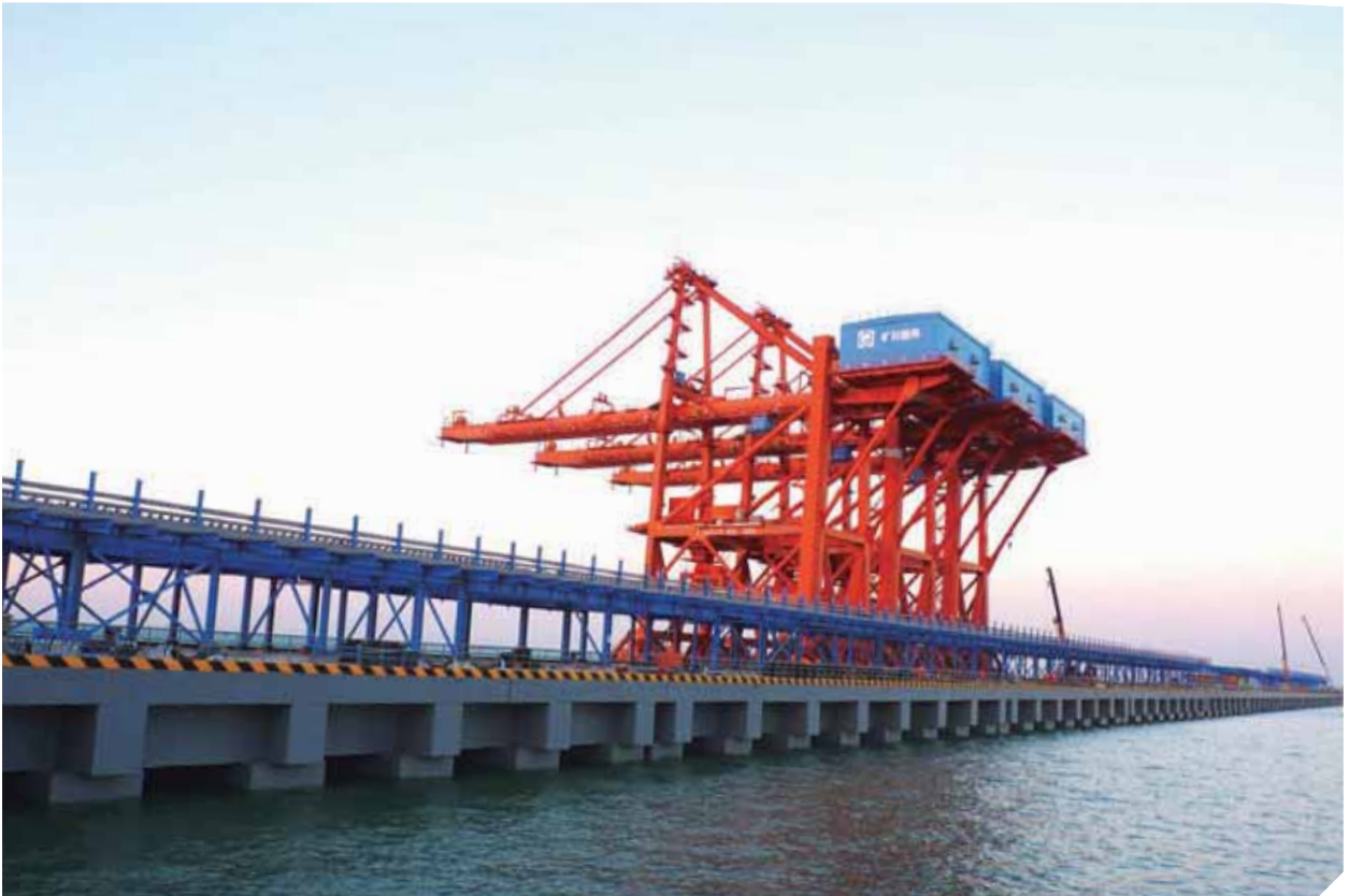
Huanghua port 200000 ton iron ore terminal project
